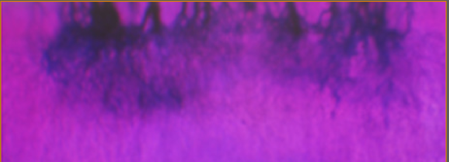
An example of insulation erosion caused by partial-discharge activity. These sites are often referred to as "electrical trees."
